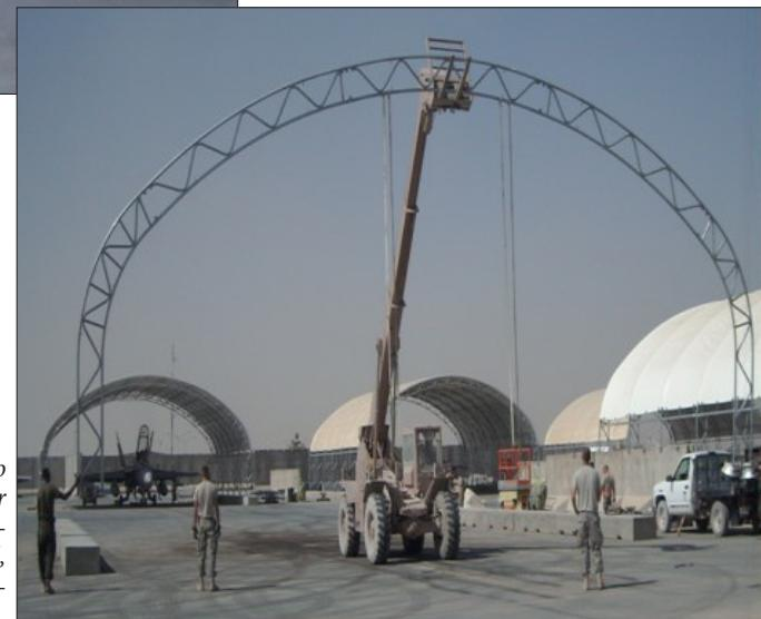
Deployed Airmen use a cherry-picker forklift to raise a part of a frame for installation at Kandahar Airfield, Afghanistan, in this undated photo. Sun-shades, like the completed ones in the background, provide shade to parked aircraft, decreasing the outdoor working temperature by as much as 30 degrees.
